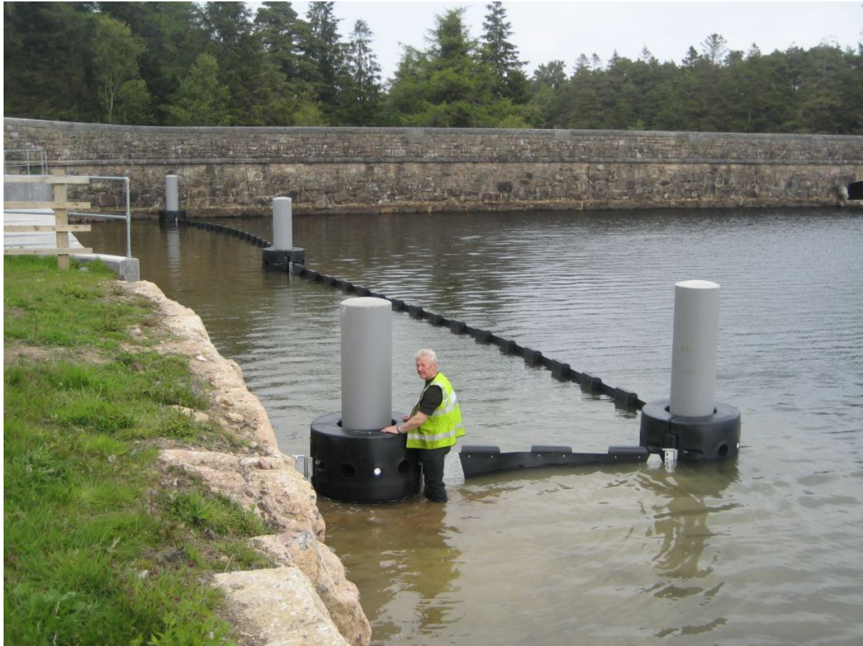
Picture of a variable water level boom.
